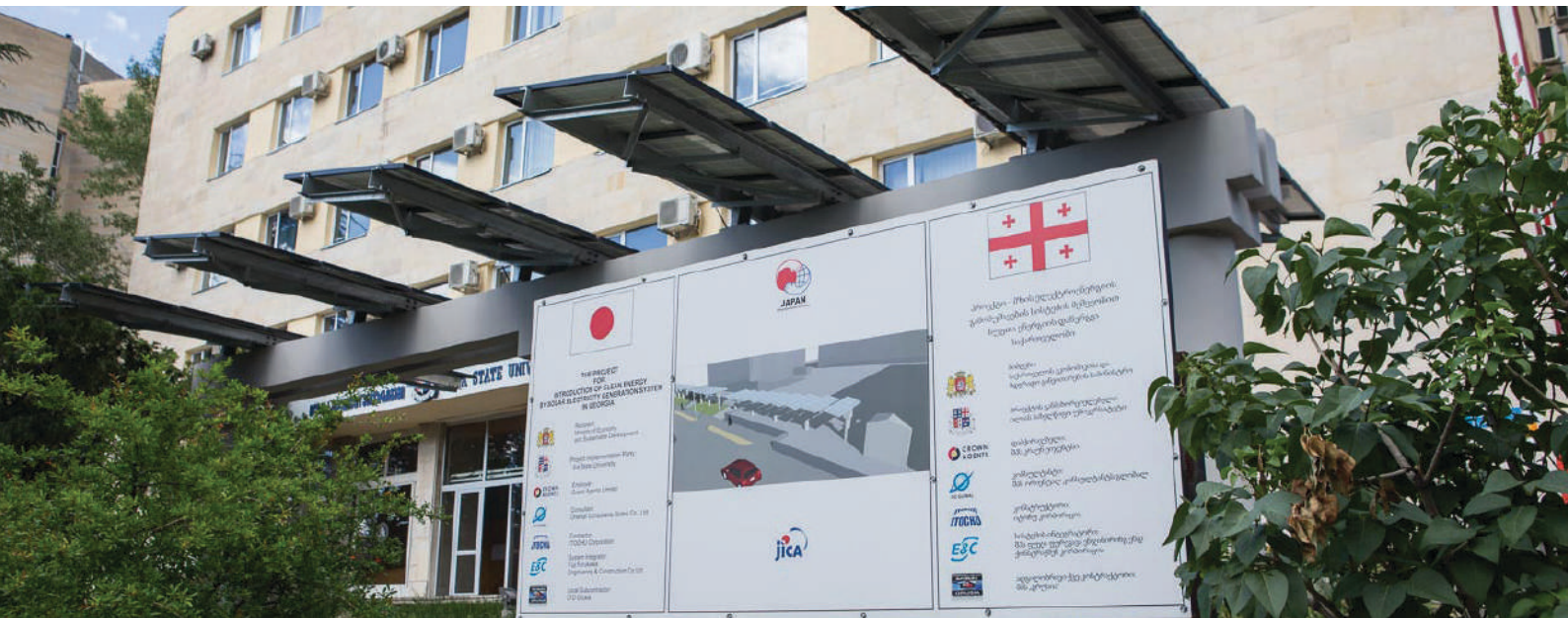
Ilia State University, Solar Photovoltaic Systems
